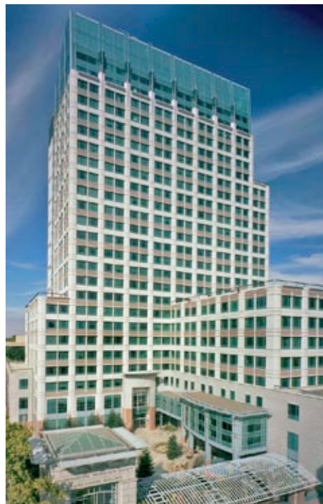
The Joe Serna Jr. Cal/EPA Headquarters in downtown Sacramento, completed in 2001, will soon undergo recommissioning. Photo: John Swain.
